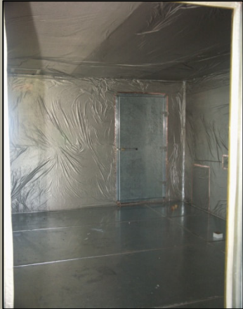
Reception and testing rooms lined with metallic fabric.
