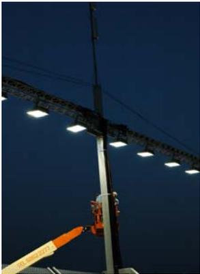
Antenna installation on a light tower
